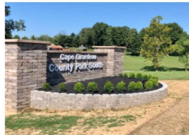
Replaced Broken Sign at Park
